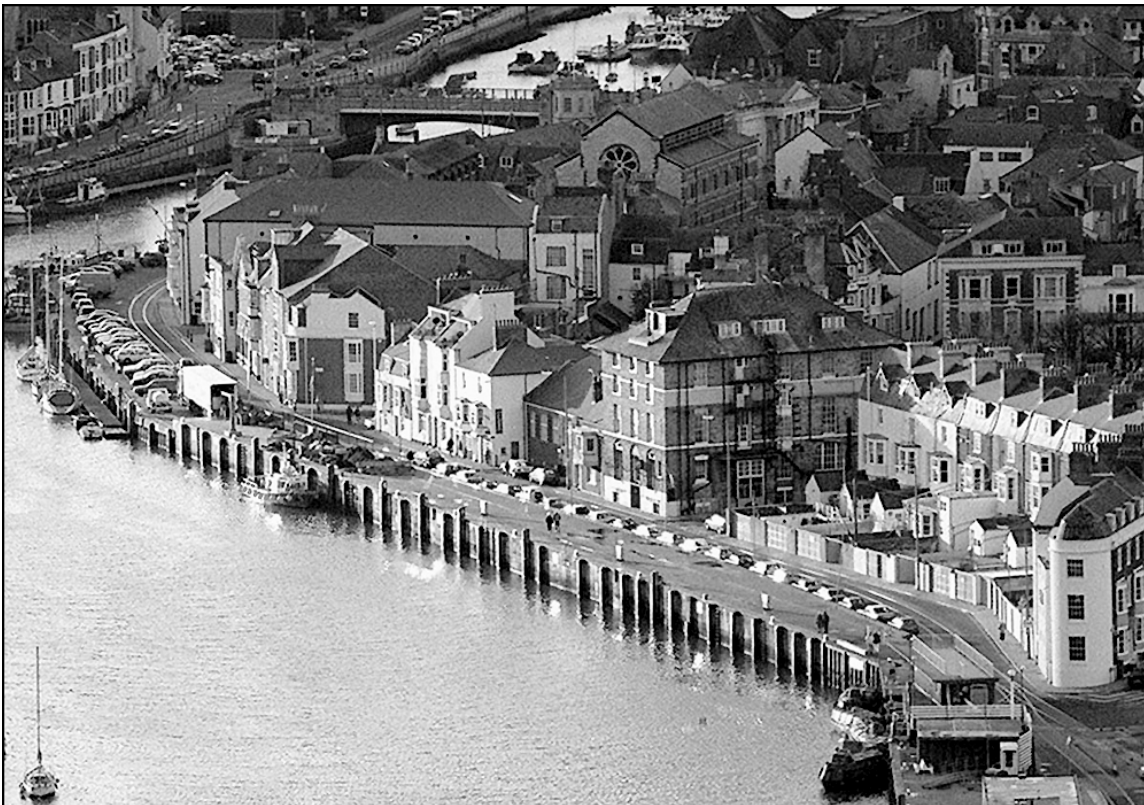
Weymouth harbour. J.I. Associates Ltd, Portland
